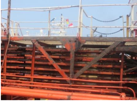
Application of 1 st coat primer
