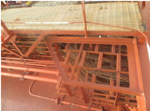
Application of 2 nd coat primer
